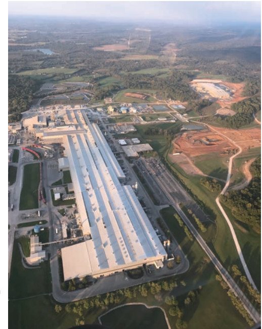
Expansion of Logan Aluminum, where 50 percent of aluminum coils for beverage cans sold in the U.S. are produced, is in progress in line with the entering of new fields.
