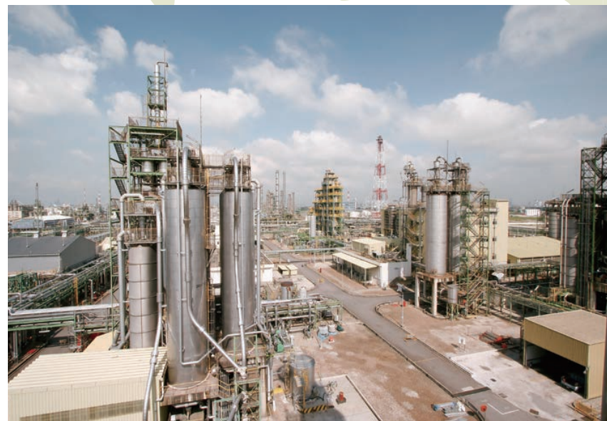
Chemical plants constructed in the 1970s on Jurong Island, currently the center of the petrochemicals industry
