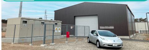
Namie Namie EV Battery Station
