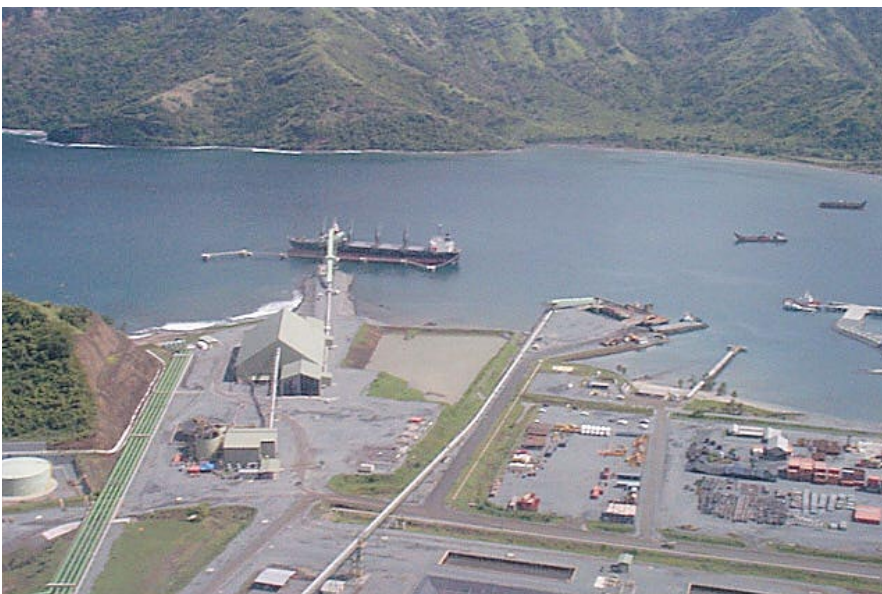
Carrying the first shipment from the Batu Hijau copper and gold mine in Indonesia, the Astro Ace left for Japan in December 1999.
