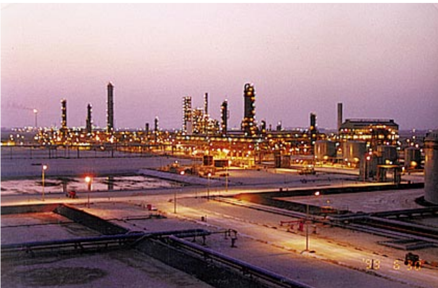
Qatar Fuel Additives Co.'s methanol/MTBE plant, for which Sumitomo undertook project finance.
