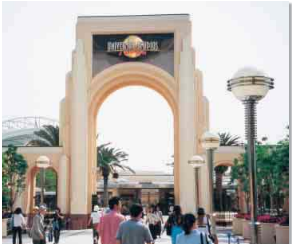
Universal Studios Japan opened in March 2001. We undertook the transportation of all its 18 attractions to the site from the U.S. and other countries, delivering them on time in accordance with its construction schedule. Universal elements, Universal Studios Japan™ & © Universal Studios. All rights reserved. CR01-3028.
