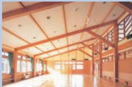
Sumisho & Mitsuibussan Kenzai Co., Ltd. constructed the structural frame of a wooden school building (multipurpose hall).
