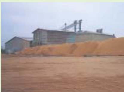
Rice husk power plant in Thailand (Roy-Et Green Power Project)
