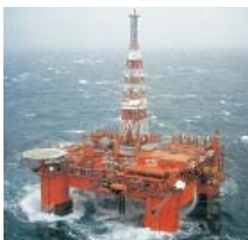
Floating Production Vessel operating in North Sea, U.K.
