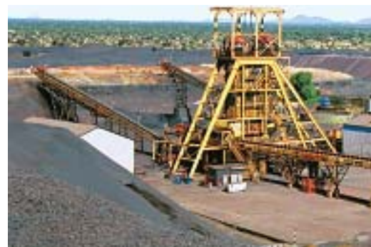
Vertical Shaft at Nchwang Manganese Mine, in South Africa
