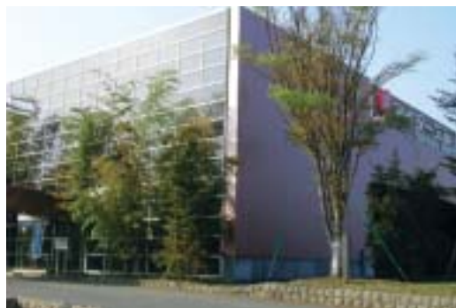
The Sagae Plant, the main plant of the top metal siding manufacturer IG Kogyo
