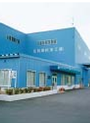
The Shiga Plant of Sumisho Steel Sheets Works, equipped with cutting-edge steel processing facilities
