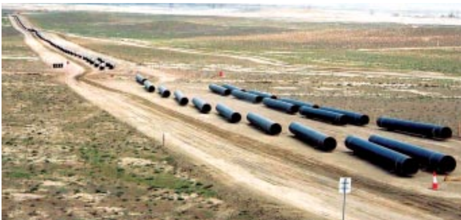
Line pipes installation site in Azerbaijan
