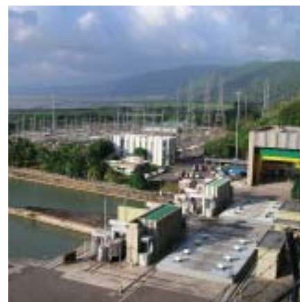
CBK Hydropower Plant in the Philippines
