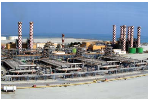
Bahrain's Hidd IWPP, for which we have acquired operating rights. We are building a new desalination plant (60MIGPD*) in addition to the existing power & desalination plant (965MW + 30MIGPD) and will carry out power & water production and operation for the next 20 years.
