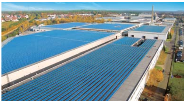
A solar power generation system installed at a Michelin factory by our system integration partner. Its power generation capacity of 2,600kW and annual power generation of 3,300 MWh are the largest in the world for the rooftop installation type. It contributes to the reduction of oil consumption for around 850kl per year.
