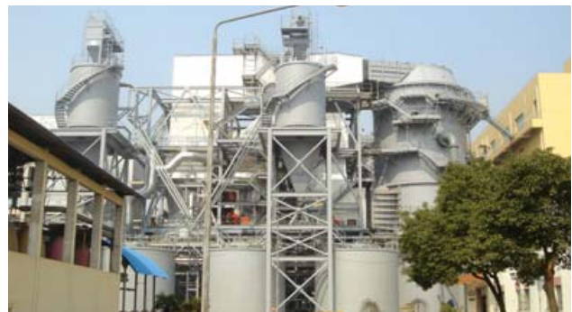
In a joint project with Ishikawajima-Harima Heavy Industries Co., Ltd., we received an order from the Shanghai Municipal Electric Power Company for a Flue Gas Desulphurization Systems for the Waigaoqiao coal-fired thermal power plant. The completed facility was handed over in May 2006. As the first Flue Gas Desulphurization plant in the Shanghai district, it is expected to reduce air pollution.
