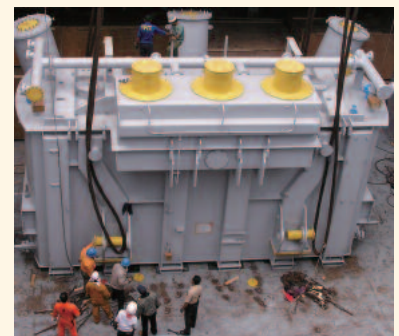
Unloading of main transformer
