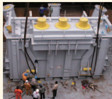
Unloading of main transformer
