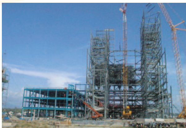
Power plant under construction (prior to work suspension)
