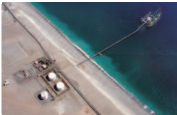
The port facilities for sulfuric acid discharging in Chile were expanded in 2007. Interacid Trading, a Swiss-based sulfur and sulfuric acid trader, possesses its own facilities and operates a trading business that is responding to the global demand for sulfur and sulfuric acid.
