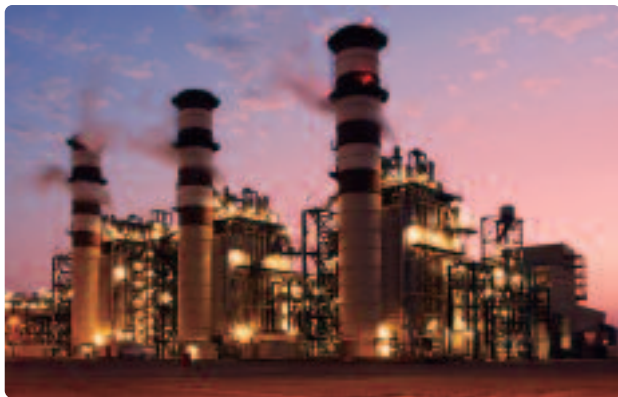
The Shuweihat S1 power plant boasts facilities capable of generating 1,500MW of electricity as well as desalinating 460,000 tons of seawater a day. Having acquired a 20% interest in this project, we offer stable supplies of electricity and water based on a long-term contract with the Abu Dhabi Water and Electricity Company (ADWEC).
