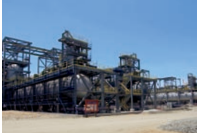
Part of the processing facility in the Ambatovy nickel project in Madagascar. Currently under construction, this project is one of the world's largest of its kind, and is expected to produce 60,000 tons of nickel metal annually.
