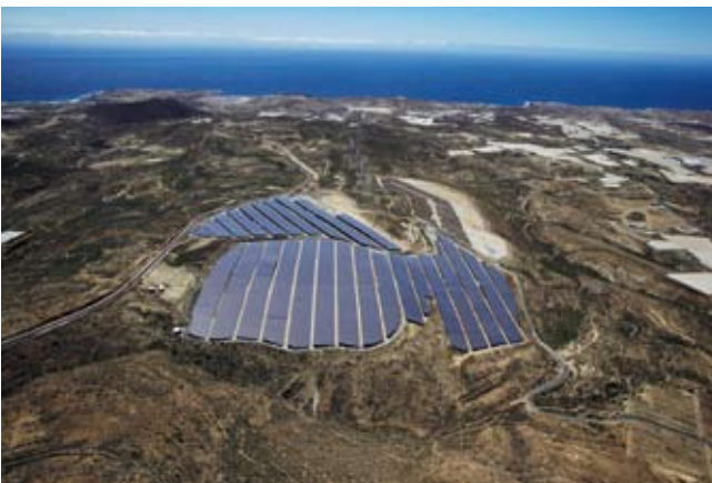
Solar power generation project on the island of Tenerife, Spain
