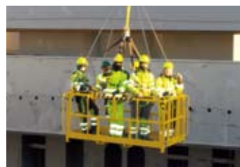
Workers wearing personal protective equipment and individual safety harnesses during vessel unloading operations—Floro, Norway
