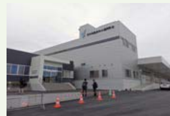
A building housing the offices for the Kesenuma Shishiori Fisheries Processing Cooperative Association and a refrigerated warehouse
