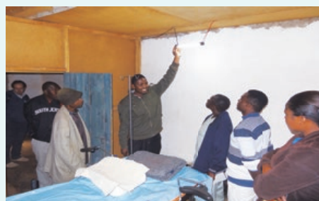
A delivery room equipped with a solar-powered light
