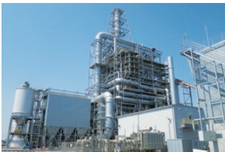
Handa Biomass Power Plant in Aichi Prefecture, Japan
