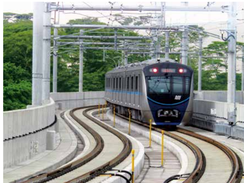
MRT railcars traveling alongside a main road in Jakarta
