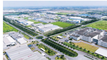
Thang Long Industrial Park (industrial park development)
