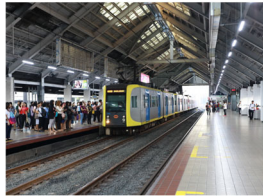
Manila LRT-1 project (railway business)
