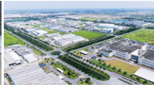
Thang Long Industrial Park (industrial park development)
