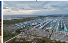
Press Metal's aluminum smelting plant (Malaysia)
