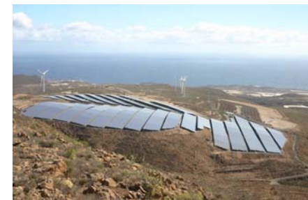
Solar power generation project in Spain
