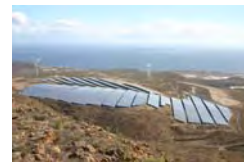
Solar power generation project in Spain
