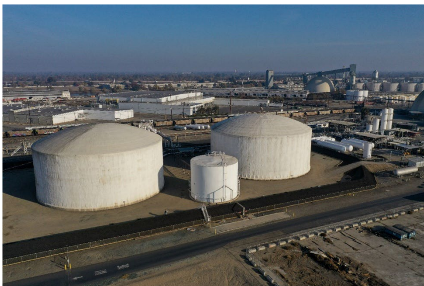
CALAMCO Ammonia Terminal in Stockton, California
