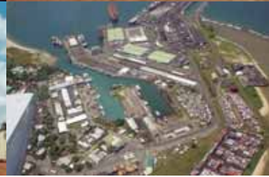
(Upper) Construction site (Lower) Toamasina Port
