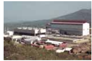
Construction of a geothermal power plant (Indonesia)
