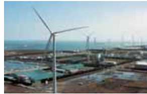
Wind power generation project (Ibaraki Prefecture)
