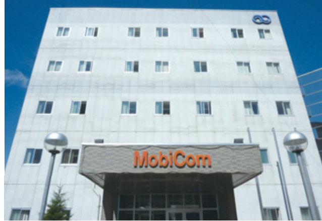
MobiCom Corporation Head Office
