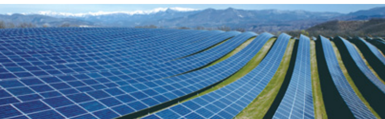
Solar power plant in Les Mées, a city near Marseilles in southern France
