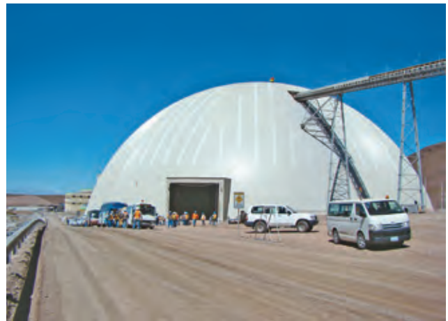
Bolivia's first dust control dome
