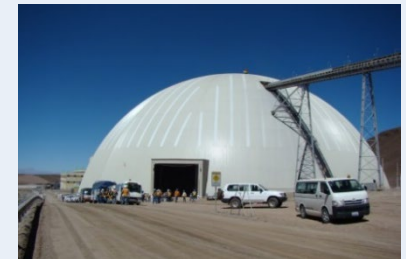
Huge dome for the purpose of preventing coal dust dispersion in the San Cristobal Mine
