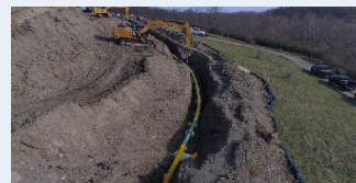
Construction site of a land pipeline
