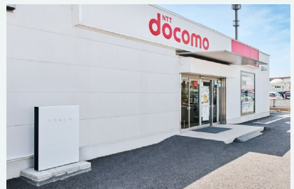
Battery chargers: the bottom left of the picture
