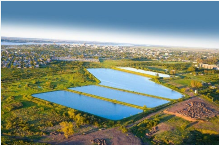
Sewage treatment plant in Rio Grande do Sul Province
