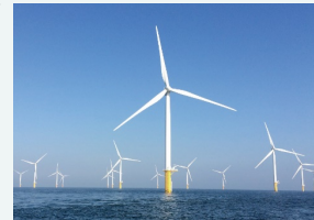
Offshore wind turbines, also known as "egrets"
