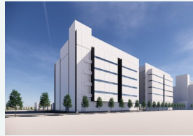
netXDC Chiba Center No. 3
