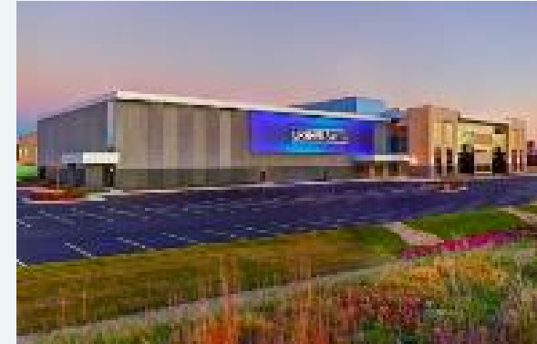
USL Head Office (Minnesota, USA)
