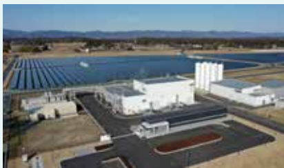
Fukushima Hydrogen Energy Research Field (Photo credit: NEDO)
