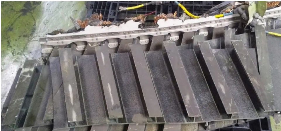
Structural components before incineration
