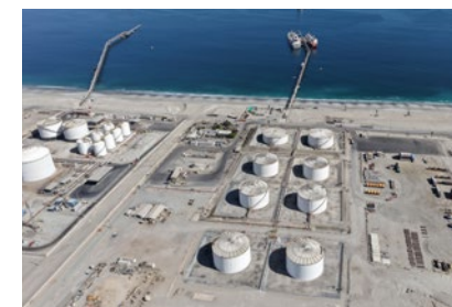
Interacid's tank terminal located in Mejillones, Chile
