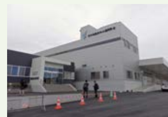
A building housing the offices for the Kesenuma Shishiori Fisheries Processing Cooperative Association and a refrigerated warehouse
