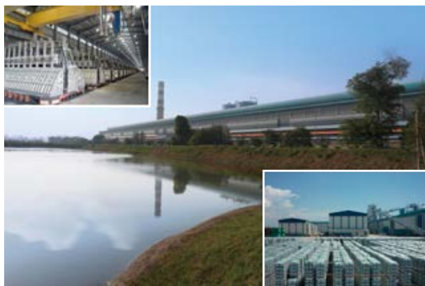
Our aluminum smelting joint venture with Press Metal, in Malaysia
