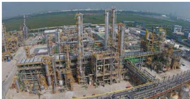
CEPSA Química China S.A.'s phenol plant in Shanghai
