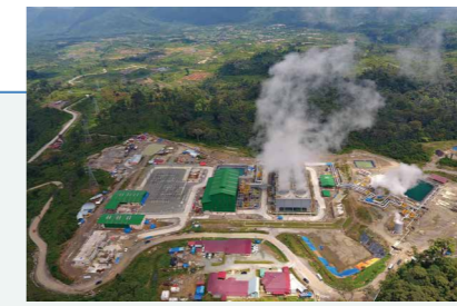
Geothermal power plant in Muara Laboh (Indonesia)
