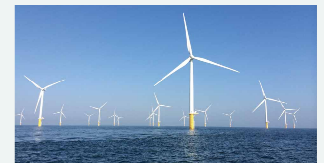
NorthWind offshore wind farm (Belgium)
