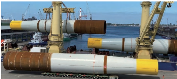
Foundation of offshore wind power generation (monopile)
