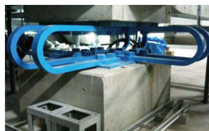
U型鋼材ダンパー U-shaped steel dampers
