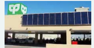
Solar panels installed on building walls
